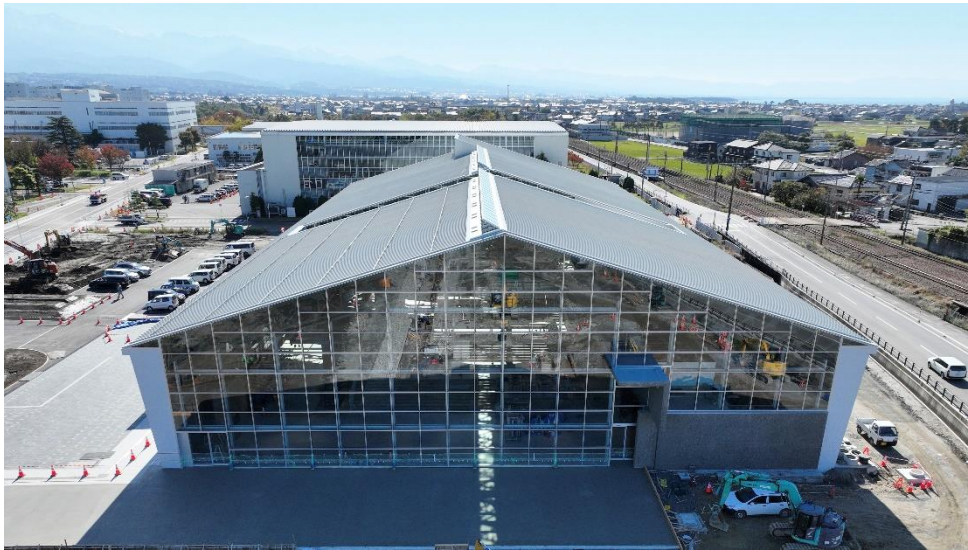
Building with a curtain wall on one side
