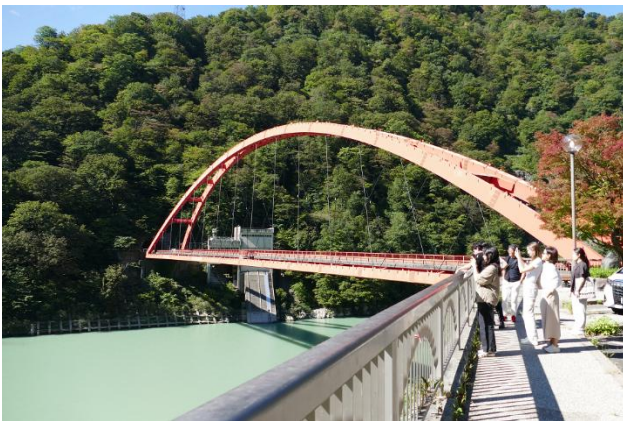
Field survey at Unazuki Dam
