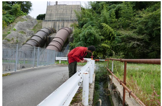
A GSD student viewing a waterway at Hokuriku Electric Power Company's Kokuto No. 3 Power Plant
