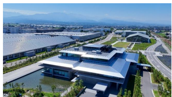
YKK AP 30 Building
