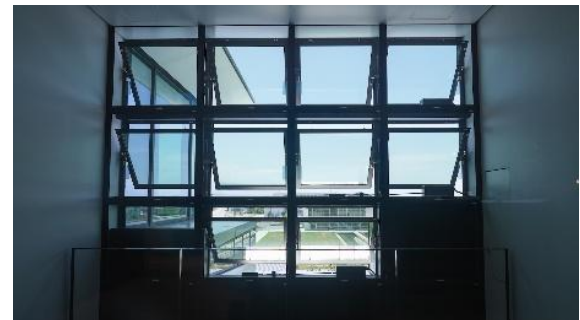
"EXIMA 31 Balance Way" windows for natural ventilation
